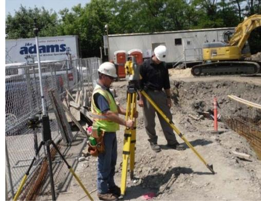
Figure 15 Robotic Total Station in the field
