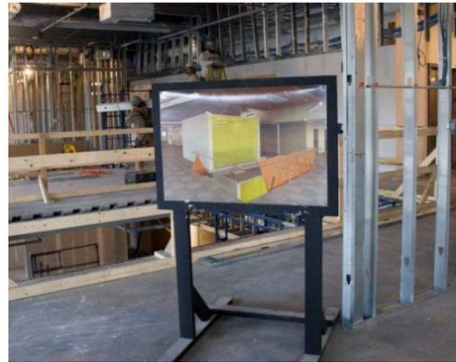
Figure 17 Interior rendering on site to guide construction
