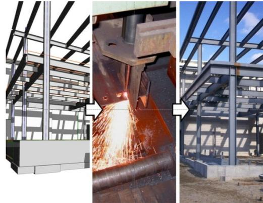
Figure 16. Fabrication model, CNC steel fabrication and erected steel
